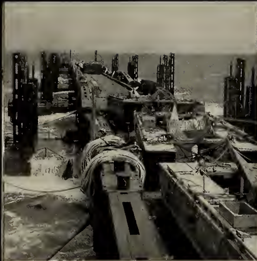
9. Extending from the pierheads to the shore were seven miles of floating roadways, over which the trucks carried the cargo into France. A section of them, 480 feet long, is shown above being towed across the English Channel.
